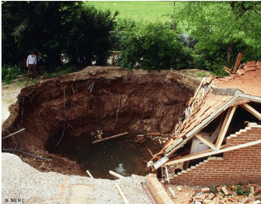
Figure 1.7 Example of subsidence in gypsum karst in Ripon, England (Cooper & Calow, 1998)
