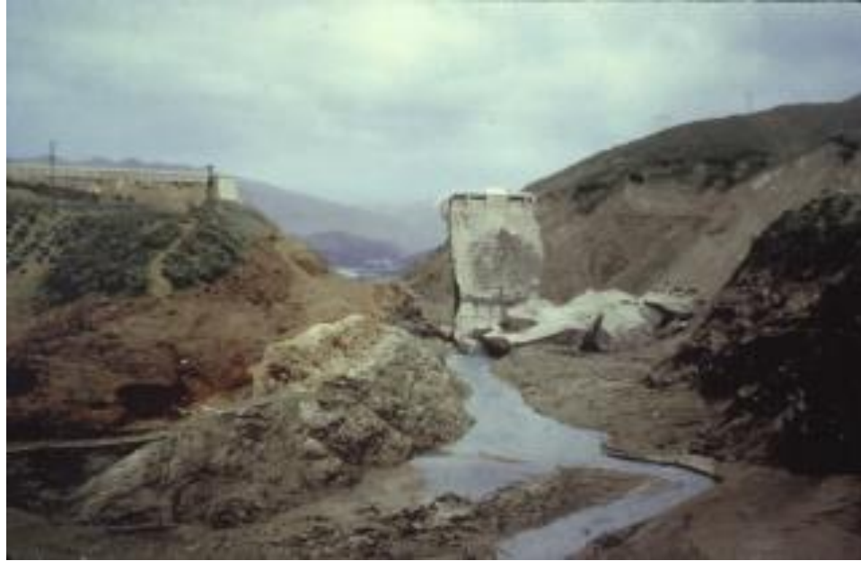
Figure 1.8 A picture of the damaged St. Francis dam in Los Angeles, 1928 (Rogers, 2007)
