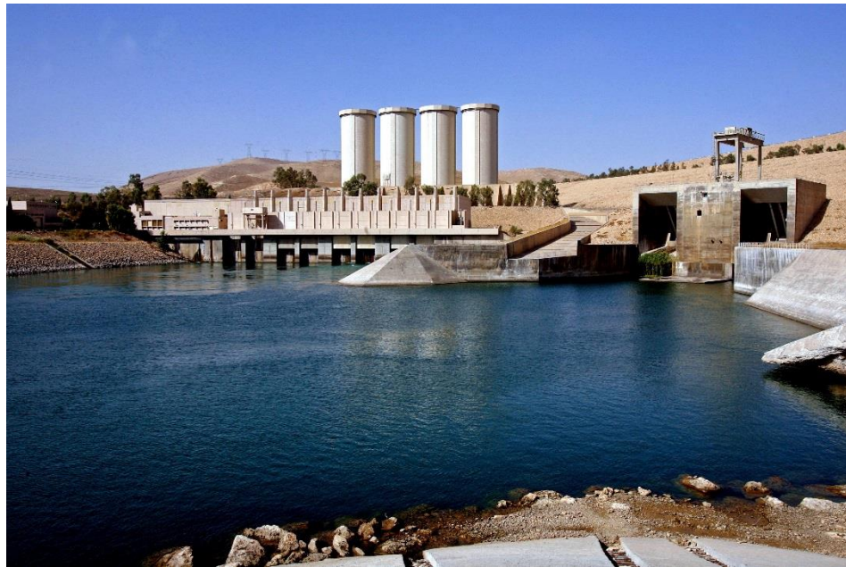
Figure 1.9 The Mosul dam in Iraq, built on a bed of gypsum rock (Hanchey, 2016)
